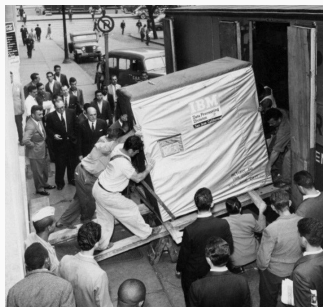
IBM 5MB hard drive (1956)
