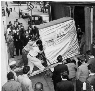
IBM 5MB hard drive (1956)
